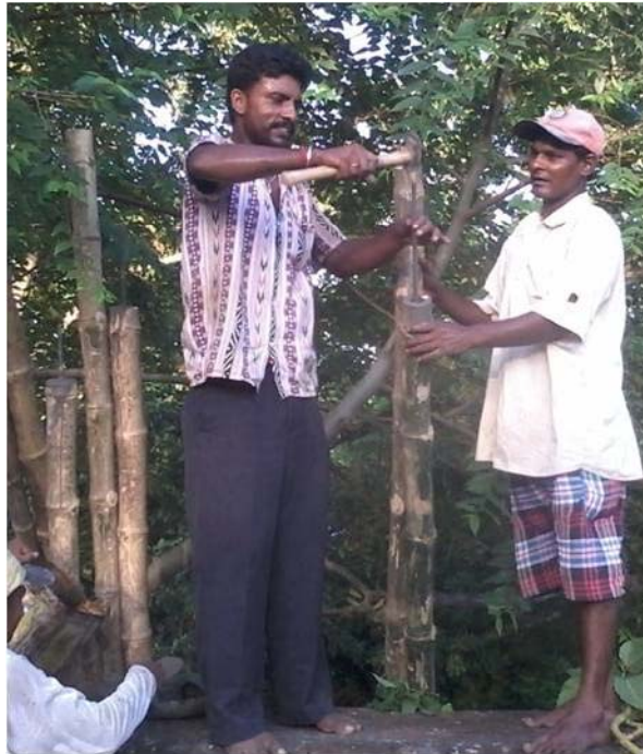
Grouting 12mm dia rods in the columns and grouting the rods-column assembly in the RCC slab
