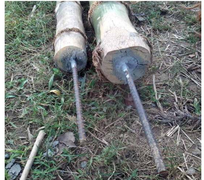
Grouting 12mm dia rods in the columns and grouting the rods-column assembly in the RCC slab
