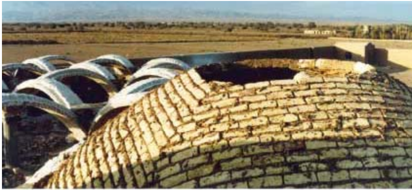
The construction of these domes is through visual estimation. High up in the dome, the 'squares' meet to become a circle.
