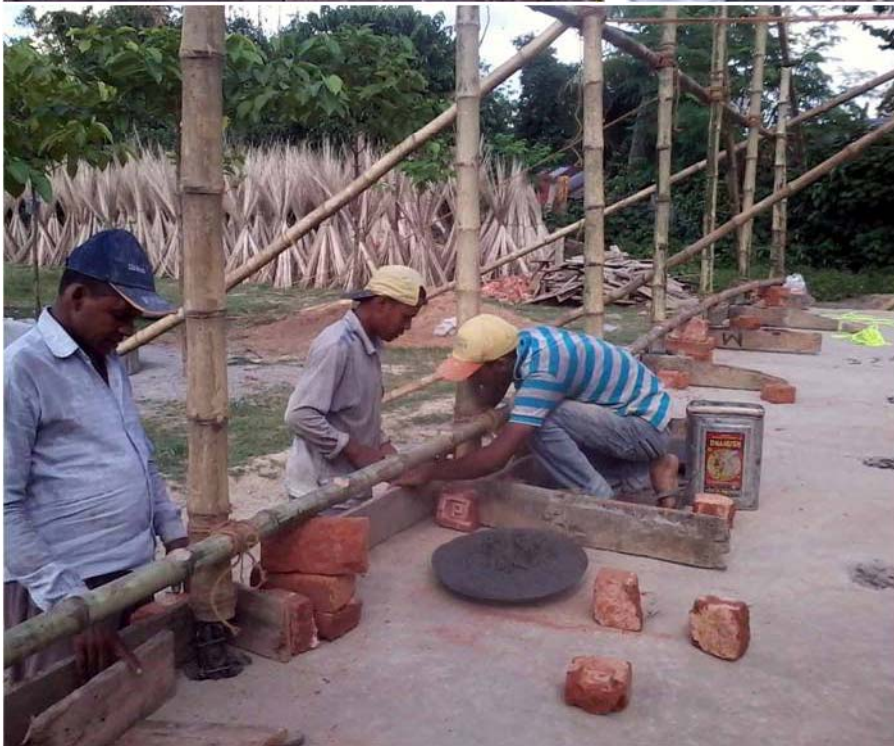
Grouting 12mm dia rods in the columns and grouting the rods-column assembly in the RCC slab
