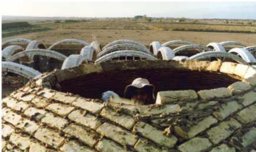
The construction of these domes is through visual estimation. High up in the dome, the 'squares' meet to become a circle.
