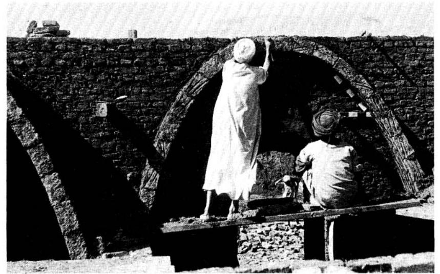
17. Masons insert dry packing in the interstices
